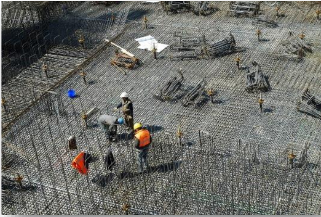
Electrical and Construction
