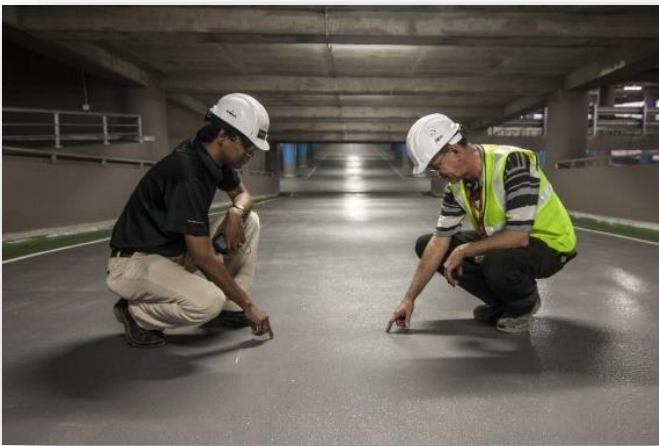
Building Inspection and Maintenance
